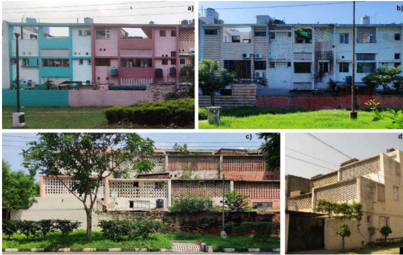
Figure 5: Rear Facades of Phase 1 Frame Controlled Houses (a,b) - Planar Facades, two and a half floors, and the presence of jaalis in patches. Rear facades of Phase 2 Frame Controlled Houses (c,d) - Recessed built forms and full-width jaalis (Gupta 2024)
