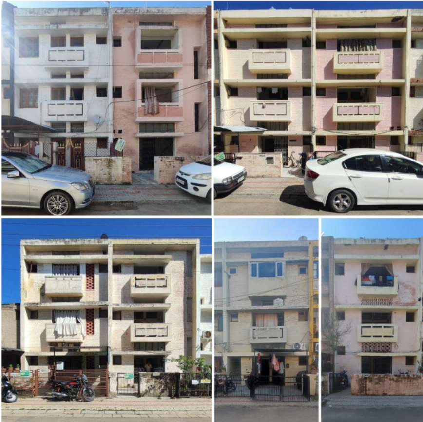
Figure 11: Front Facades in Phase 2 (Sector 35) - Most houses have a similar built profile under the frame control, with a central balcony and verandah and two smaller windows on the sides. The play is visible in the brick jaalis and the facade's color (Gupta, 2023)
