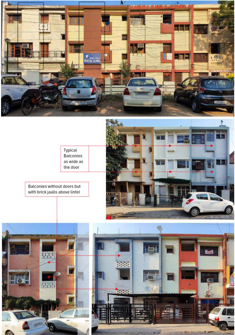
Figure 10: Houses from Sector 22 show similar house facades based on frame control clauses. (Gupta, 2021, 2023)
