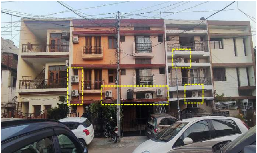
Figure 13: Houses under Frame Control in Phase 2 show water tanks and AC installations on the facades. In some cases, the windows also have desert coolers.
