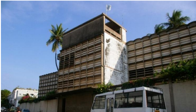
Figure 3: Golconde's regularly subdivided facade with movable louvers (Photo Courtesy: Smita Dalvi)
