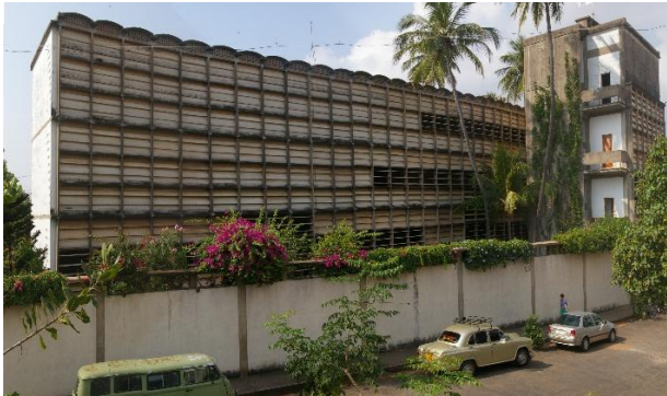
Figure 1: Golconde Dormitory in Pondicherry (Photo Courtesy: Smita Dalvi)
