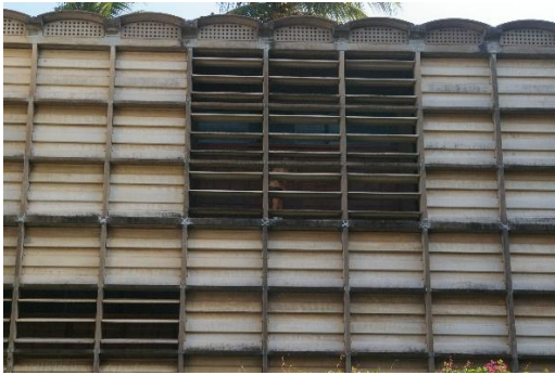
Figure 9: Golconde's custom made louvers (Photo Courtesy: Smita Dalvi)
