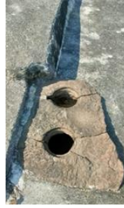
Figures 7,8,9: Underground tunnel, pressure tower and terracotta pipes at Ramlinga Talab
