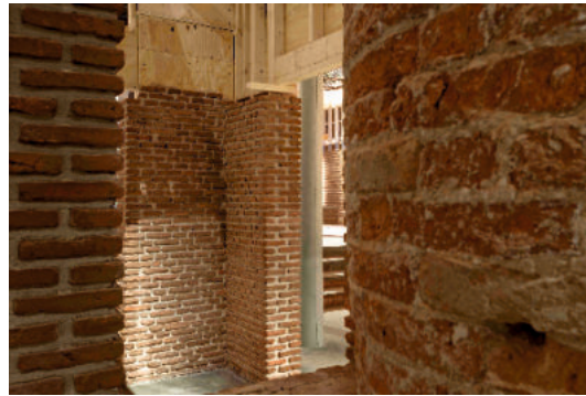
Figure 4: Ancient Italian brick masonry in lime mortar in dialogue with contemporary brick masonry made of still-in-use ancient Achakul bricks in lime mortar, establish common ground between the apparently diverse geographical and material cultures
