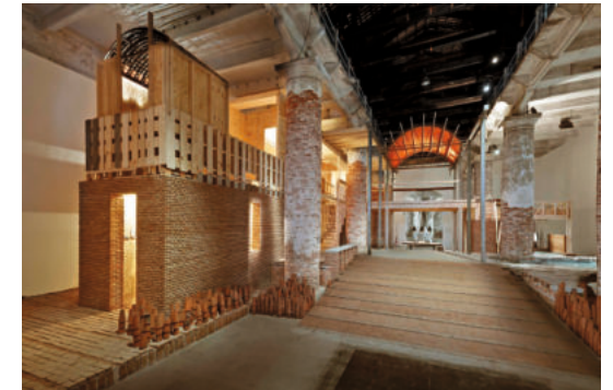
Figure 2: Seen from the rear end of the exhibition room, a ramp leads to the raised central space under the terracotta vault. Seen in the foreground is a variation of the vault system made with interlocked wine bottles above the bathroom area.
