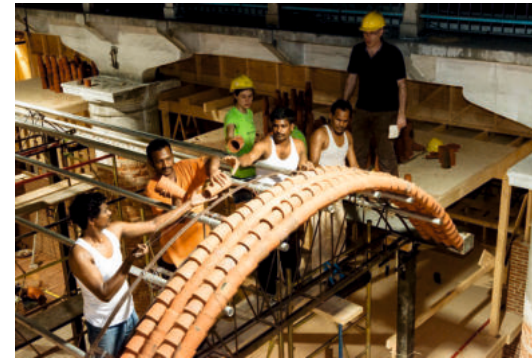
The central roof vault is made of self-supporting and interlocked, handmade terracotta tubes arranged along a catenary curve.
