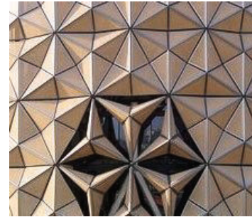
Figure 23: Façade of Al-Bahar Towers, Abu Dhabi. Source: archdaily.com
