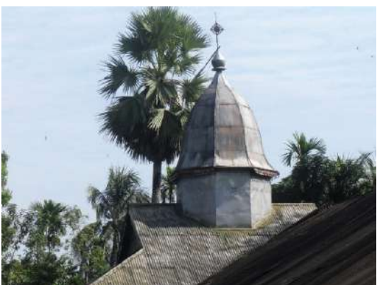
Figure 13: Spire clad in copper sheet, Namghar, Dokhinpat Satra
