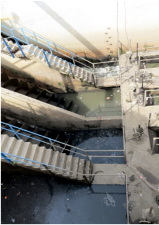
Figure 3: Screw pump at Konia pumping station that lifts wastewater to the pipe leading to the Dinapur treatment plant.
