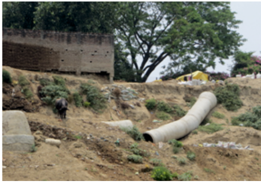
Figure 5: Broken sewage pipeline extending from Nagwa pumping station. Taken on June 2014 by Kelly Alley.
