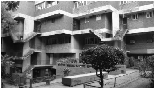
View of Tara Apartments
