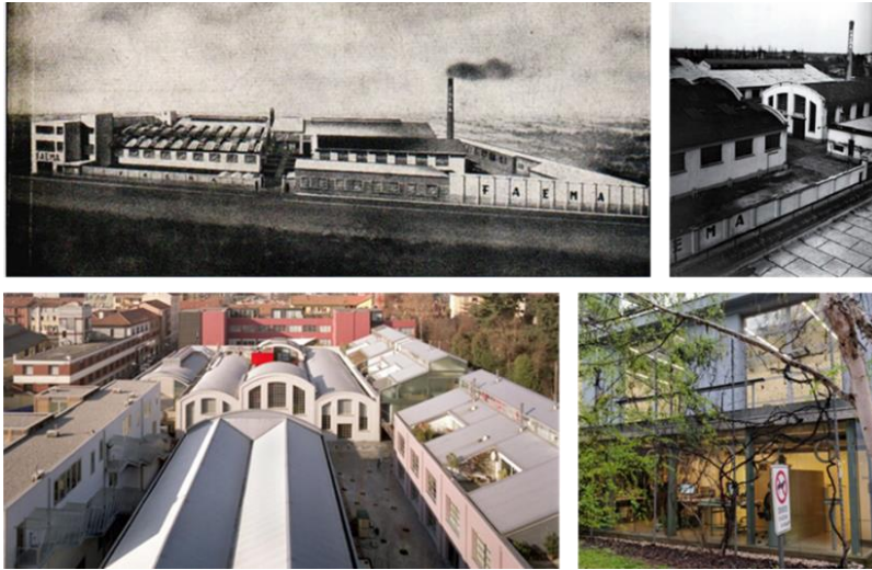
Figure 11: Transformation of the Faema Industrial Estate (L-R): Faema factory complex in 1952; Vaulted arches and compound walls (source: cafeoblog.wordpress.com/tag/via-ventura/ ); Transformed Faema factory complex in 2003 (source: Lambrate Design District); Introduction of skylights and glass walls to accommodate office and co-working spaces
