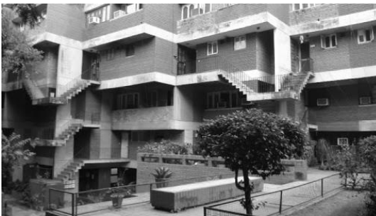
View of Tara Apartments
