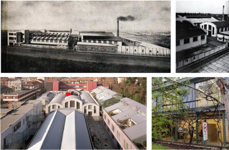
Figure 11: Transformation of the Faema Industrial Estate (L-R): Faema factory complex in 1952; Vaulted arches and compound walls (source: cafeoblog.wordpress.com/tag/via-ventura/ ); Transformed Faema factory complex in 2003 (source: Lambrate Design District); Introduction of skylights and glass walls to accommodate office and co-working spaces
