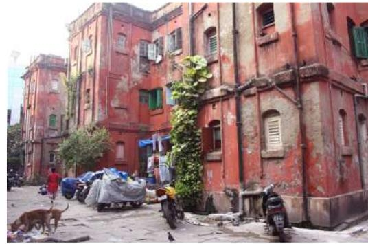
Figure 12. Damaged walls with vegetative growth
