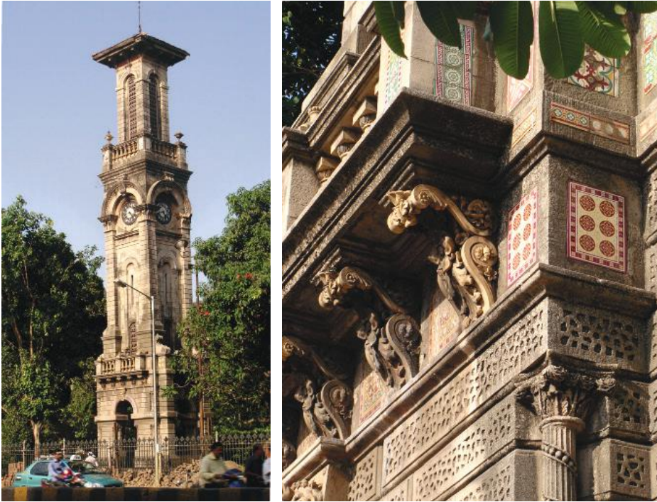
Figure 9: Clock Tower at Victoria Gardens (Now Jija Mata Udyan), Bucculla, Bombay.
