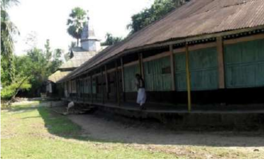
Figure 11: Mud plinth of Namghar, Dokhinpat Satra
