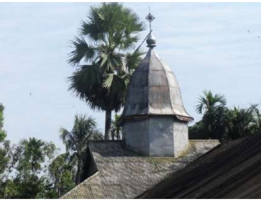
Figure 13: Spire clad in copper sheet, Namghar, Dokhinpat Satra
