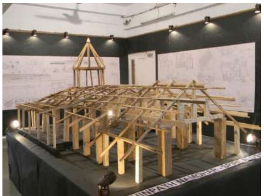
Figure 16: Model of Post and Lintel timber construction of Dokhinpat Namghar, Credit: KRVA Students' work 2010
