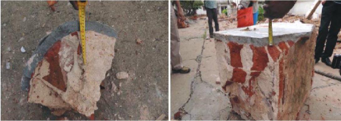
Figure 4: Load bearing masonry wall portions from the debris showing thick cement plaster. (Image Credits – NCSHS, IIT Madras)
