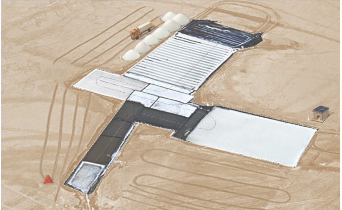
Figure 7: Salt Pan of 10 acres with the dwelling and salt collected in heaps
