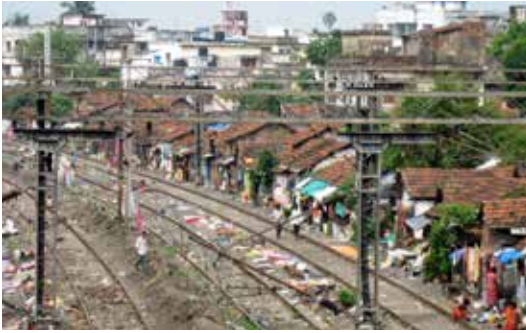
Figure 3: Slum along a railway track
